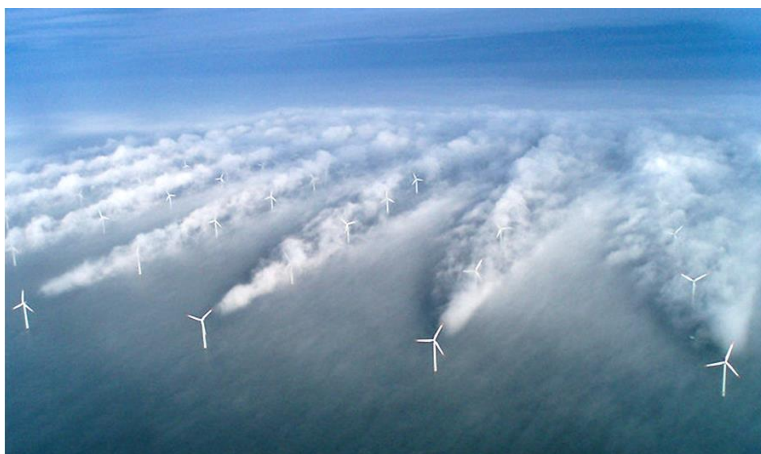
Fig. 2: Photograph of the wake interactions in Horns Rev wind farm. (Retrieved from: C.B. Hasager, L. Rasmussen, A. Peña, L.E. Jensen, P.-E. Réthoré, Wind Farm Wake: The Horns Rev Photo Case. Energies, 2013.)
